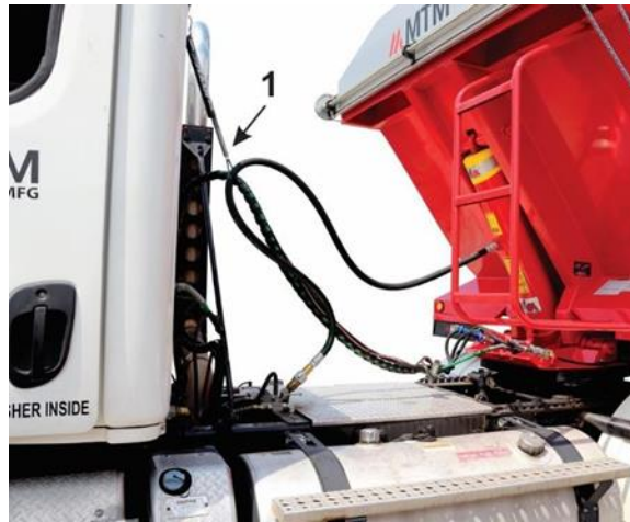
(1021) Figure 4-11 – Properly Supported Air and Brake Lines
